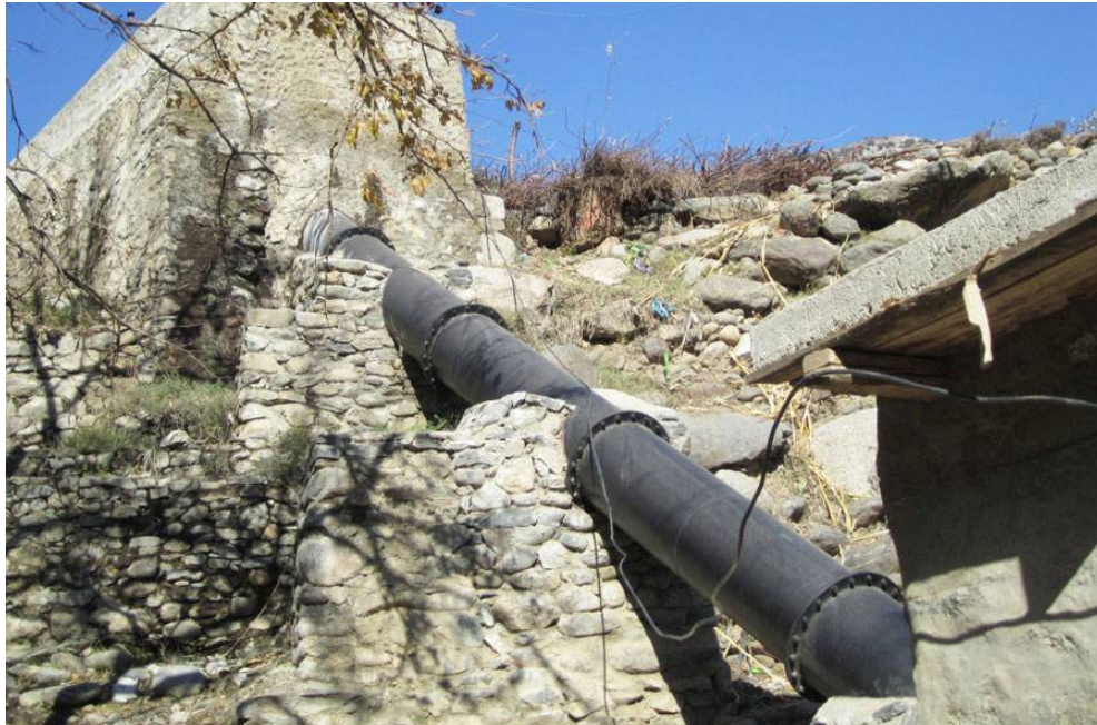
Figure 6: Forebay with Penstock
