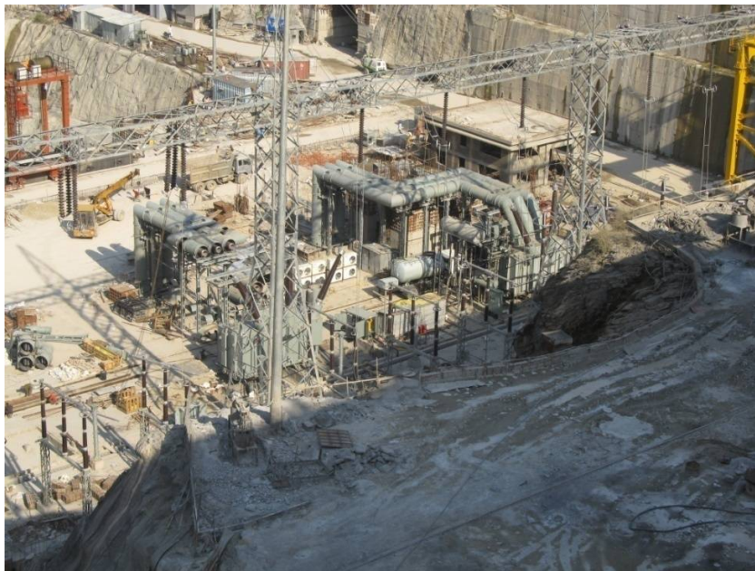
Figure 13: A switchyard under construction
