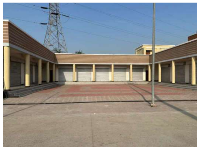
Newly Constructed Shop Complex inside Hall Premises
