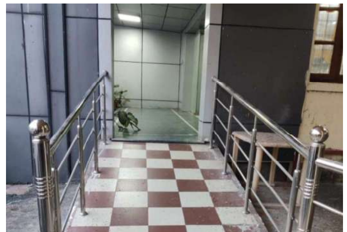
Ramps at Entrances for Differently-abled Persons
