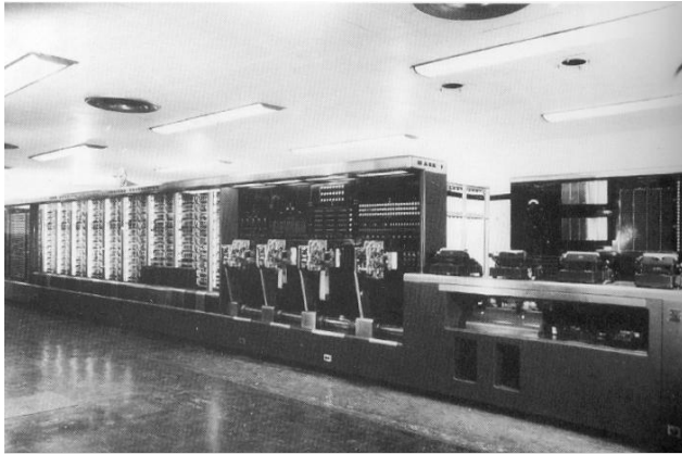
1940 - Harvard MarkI Electro-mechanical computer – 5 tons, 8 x 51 feet and 500 miles of wire
