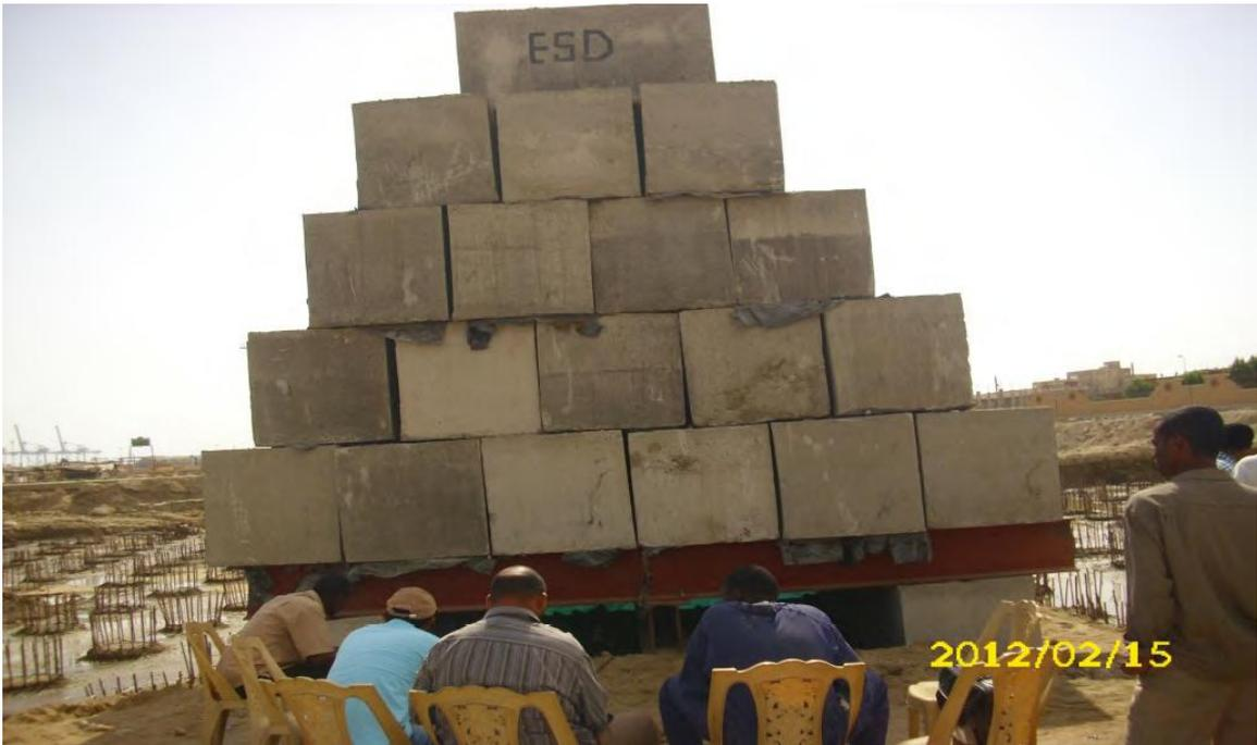
Figure 40.4 : Static Pile Load Test
