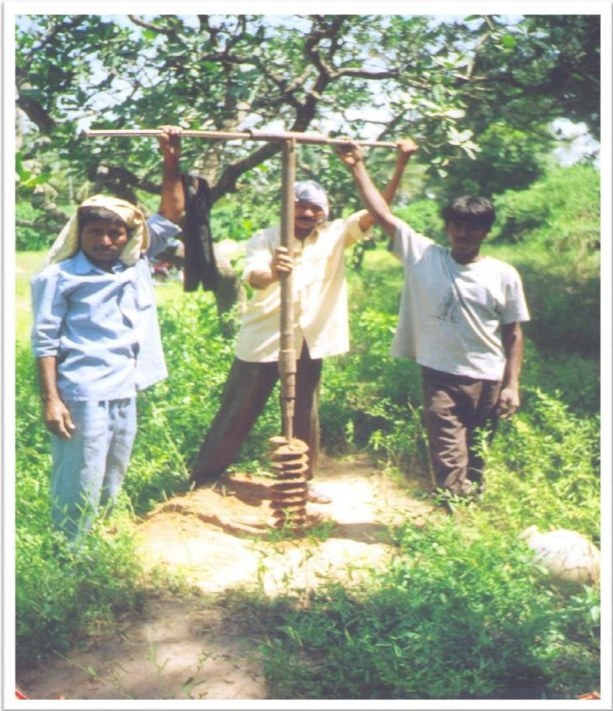
**Fig. 17.2 Manual auger boring**
