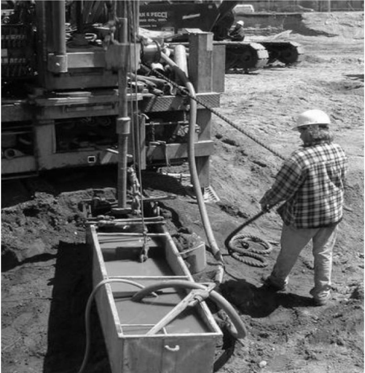
**Plate 21.1 Standard Penetration testing**
