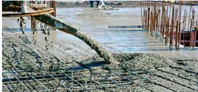
Fig: Self Compacting Concrete (SCC)
